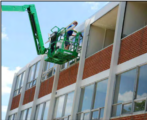
New windows are being installed in Deming Hall.
